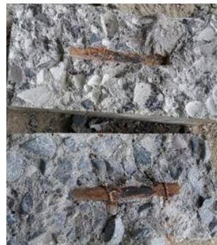
Fig. 4. Removal of embedded steel bar in concrete.
