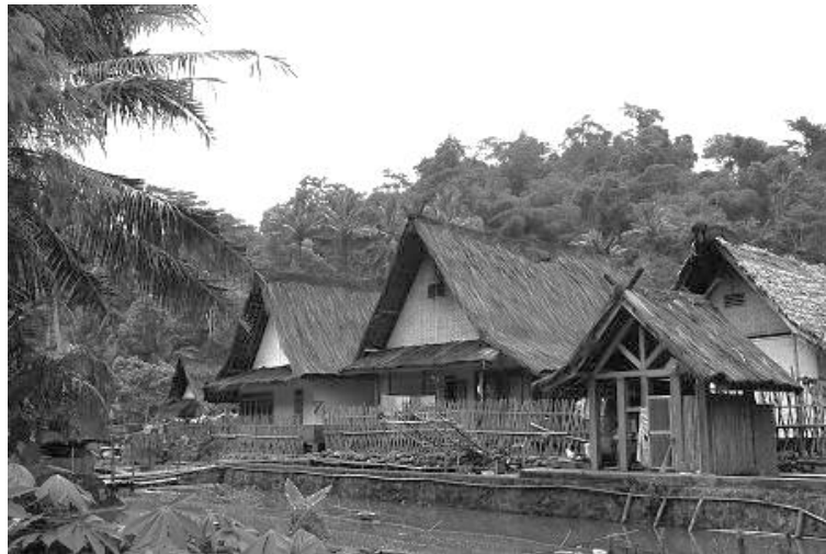
Figure 6. Cagak Gunting and Julang Ngapak Roof Type in Kampung Naga House Source: (Disparbud, 2011)
