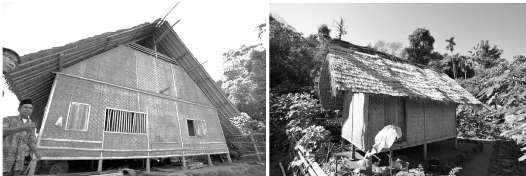
Figure 1. Sundanese House Material at Kampung Dukuh Source: (Disparbud, 2011)
