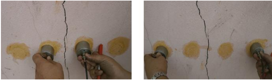
Fig. 1. Measuring crack depth by UPV.
