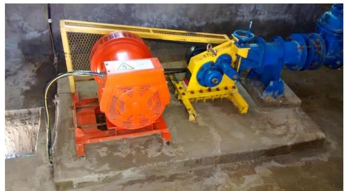
Figure 4: A micro-HEP turbine (blue, yellow) and generator (orange) located in Bario, Sarawak.
