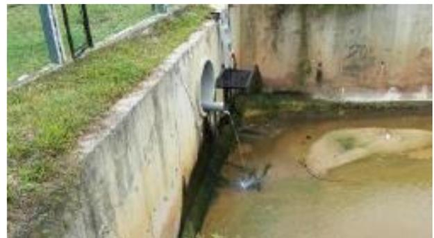
**Figure 6** The constant flowing water from effluent STP process, location at Nilai Northbound RSA, 375 PE (Courtesy by D'Bumi Water Sdn Bhd)
