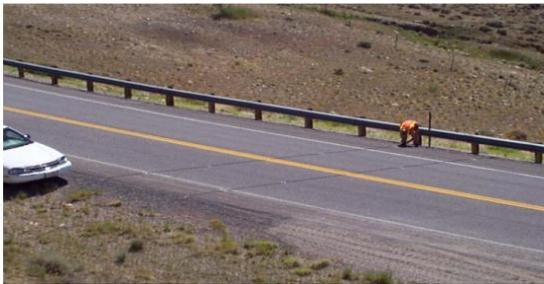
Figure 6 Road tubes on two-lane highway[55].
