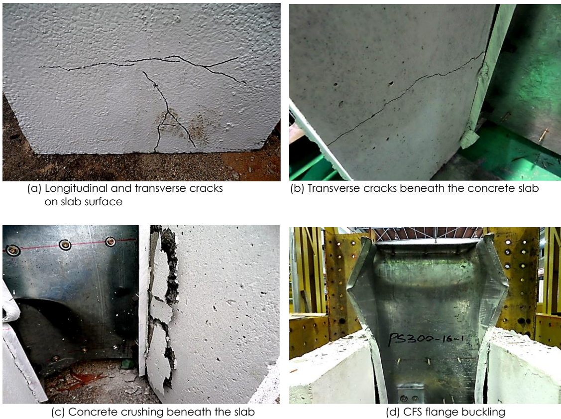
Figure 6 Failure modes of push-out test specimens
