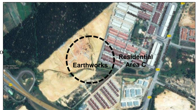
d) Taman Kempas Utama (earthworks)
