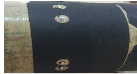
Figure 7 External flaws simulated on the pipe surface
